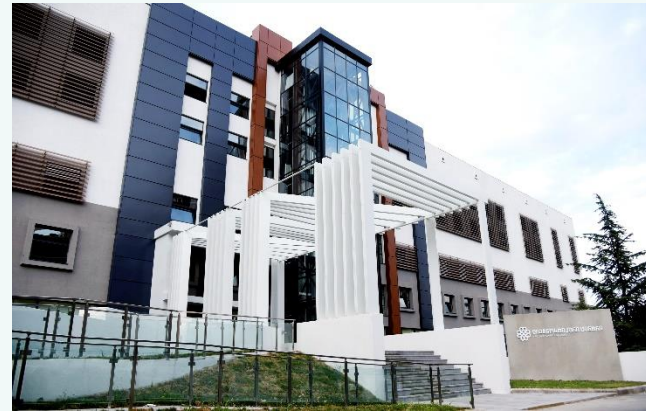
After Renovation October 2017
